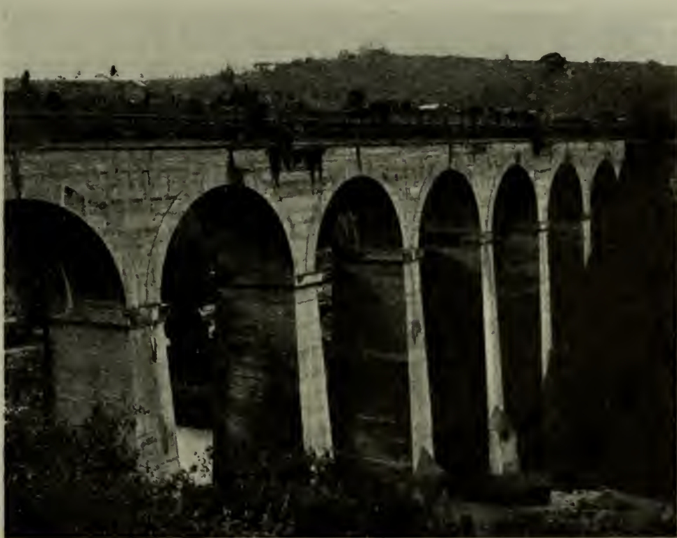
FIG. 2.—UMHLATUZAN RIVER VIADUCT, COMPLETED.
